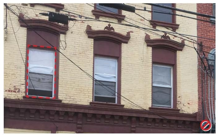
Do not replace upper floor windows with undersized vinyl replacements. Provide upper floor tenants with windows sized to the original openings.
