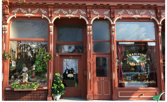
Original steel columns and cornices can be uncovered and restored to provide authentic character to a
