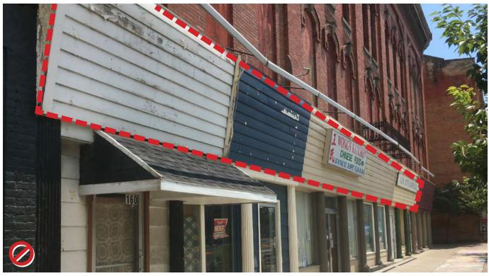
Do not cover original materials such as masonry or wood cladding with inappropriate materials such as stone veneers or vinyl siding. Do not cover up original storefront openings and details.
