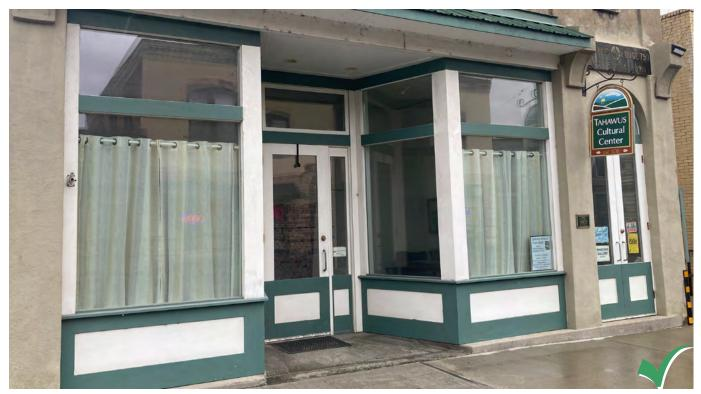
When rebuilding storefronts, utilize materials that simulate the original. Maintain original window opening sizes and transom heights.
